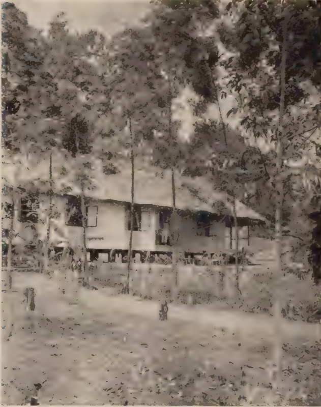
421. A B.M.S. HOUSE BUILT ON PILES (BOPOTO, NORTHERN CONGO)
